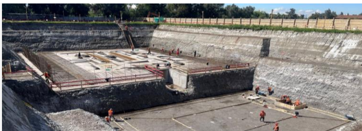
Drilling at Carabineros facility
