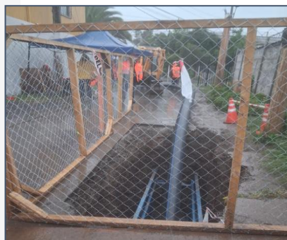
Sewage Network Renewal
